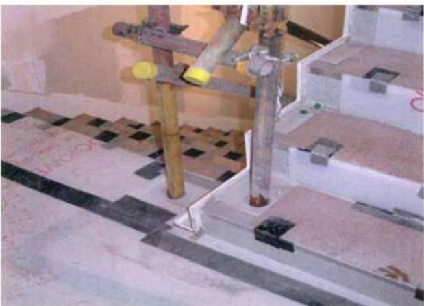
This photo shows cast sockets along the open side of a stairway, The sockets make it convenient to install temporary or permanent guardrails.
