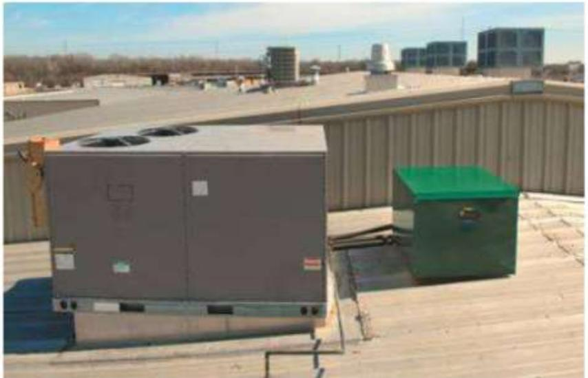
This photo shows equipment located on a roof. Positioning equipment at least 15 feet back from the roof edge will reduce the risk of falling when installing and servicing the equipment
