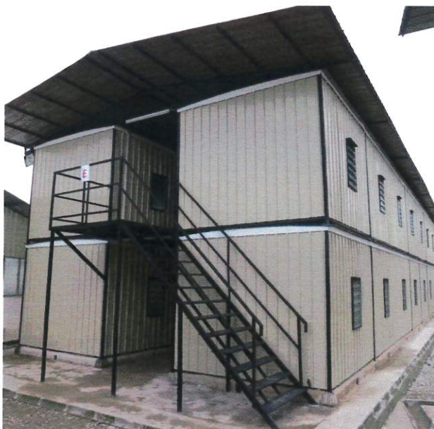
Foto 5 : CLQ Tanjung Bin Power Plant, Pontian, Johor
